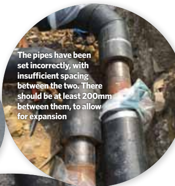
Pipes laid over existing low-voltage cables and ducts; one duct has had a section removed because the live cable had insufficient slack to permit the pipes to be laid. A minimum gap of 100mm should be allowed between crossing services
